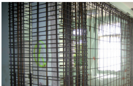
Renforcement parasismique - © Vincent Courtray - MEDDTL
